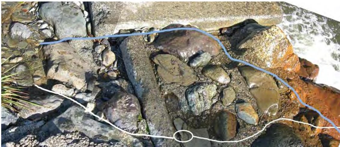
Figure 7. Two options for connecting the back-feed splash zone below the Maitai South Branch weir with the water upstream on the true right of the river. Option 1: Cut new flow path, approximately following blue line. Option 2: Pump water to approximately position of oval, and let water spill back both directions from this point, approximately following white lines.
