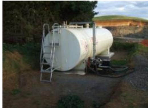
Figure 10-1 Site fuel tank with bunding to contain fuel in the event of a spill
