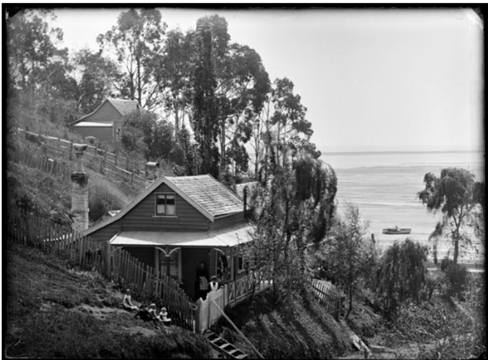
Former Johnson/Atkinson house (foreground, built before 1870) at 16 Fountain Avenue (31649, Nelson Provincial Museum)
