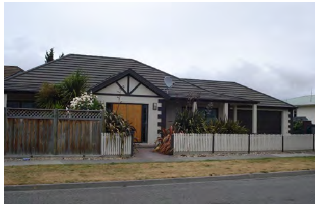
FIG 9: Example of an acceptable outcome for front fences on Classified Streets, consisting of a combination of lower (approximately 1.2m) and higher (up to 2m) elements.
