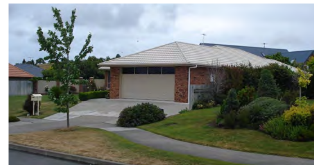
FIG 3: This triple garage set forward from the rest of the house, combined with a large paved area for parked cars does not contribute to the kind of streetscape that the Council is after.
