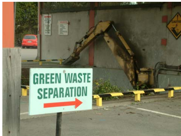
Fig 8 Pascoe Street Transfer Station Greenwaste hopper
