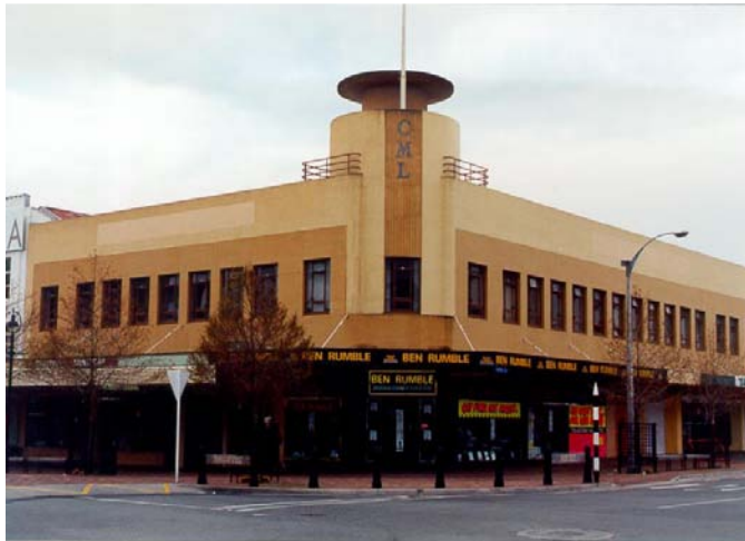
Good and bad examples of corner buildings...
